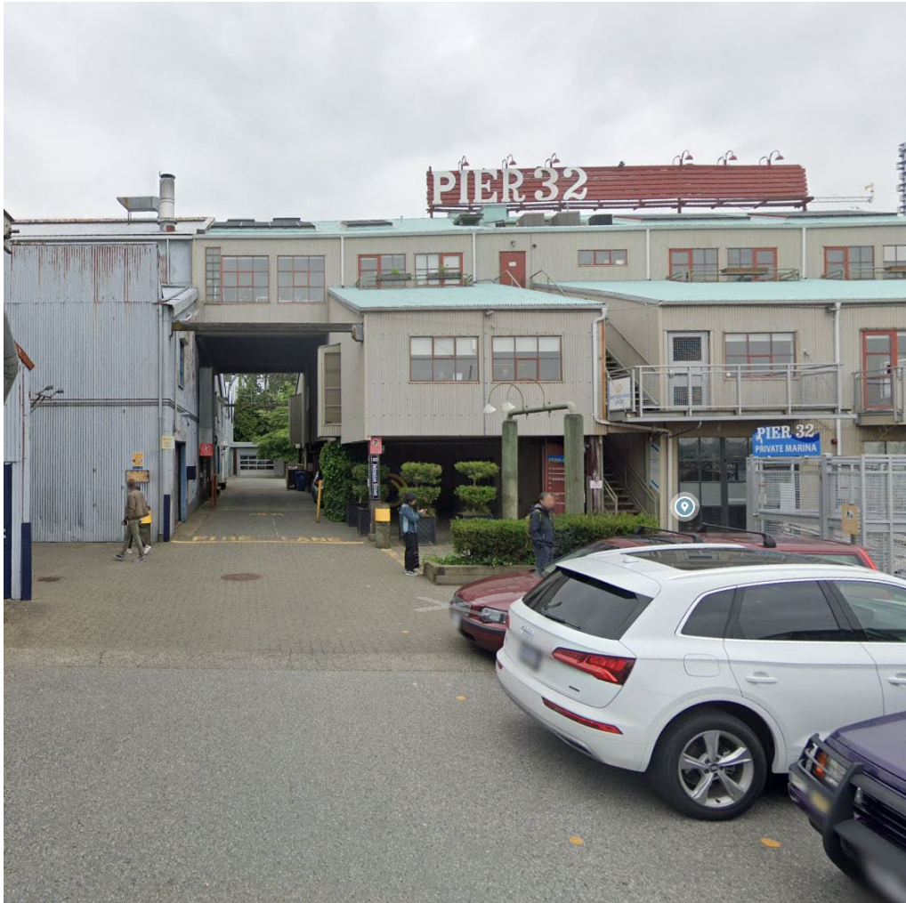
Photo 9: Pier 32 - Connected to building at 2 nd level (outside of scope of this RFEOI)
